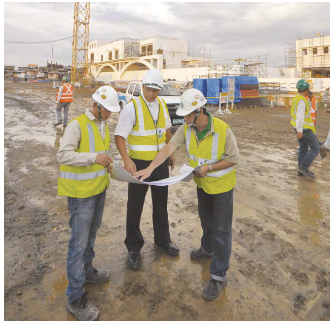
Manila Water engages local contractors in building its water infrastructure
