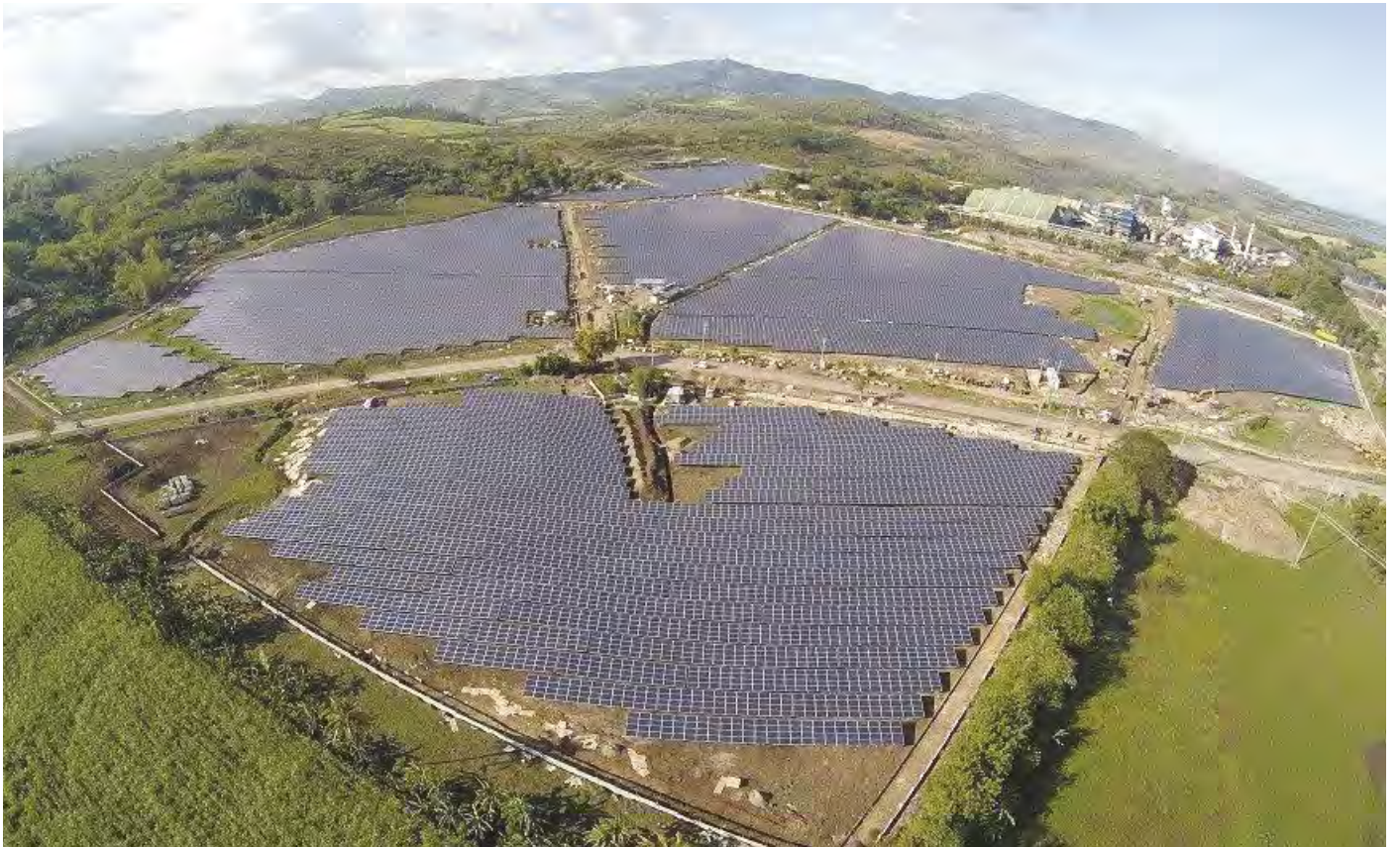
Completed site of Montesol Energy in Bais City, Negros Oriental
