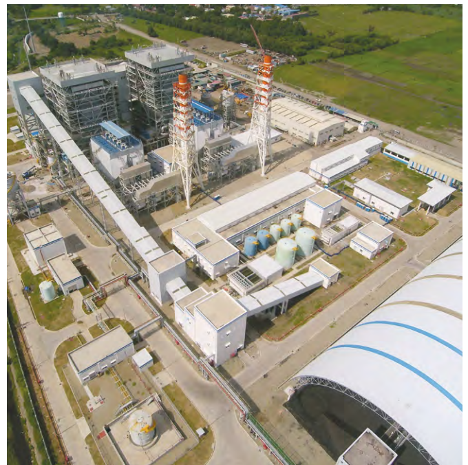
SLTEC Power Plant in Calaca, Batangas started operations in April 2015
