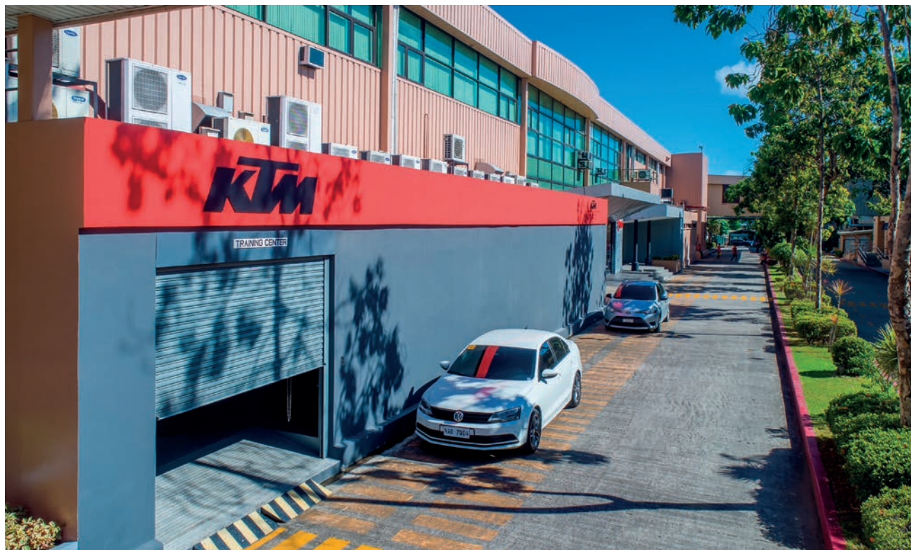
KTM’s manufacturing facility in Sta. Rosa, Laguna, in operation since 2017 as a joint venture between AC Industrials and KTM AG, now produces a variety of KTM and Husqvarna models for the Philippine market and for export to Southeast Asia and China.
