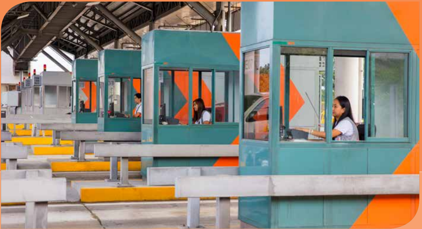
MCX helps alleviate traffic congestion along Daang Hari, Cavite, and Commerce Avenue, Muntinlupa.
