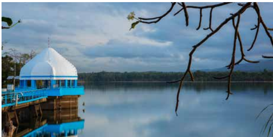
The La Mesa Dam supplies the majority of Metro Manila's water supply.
