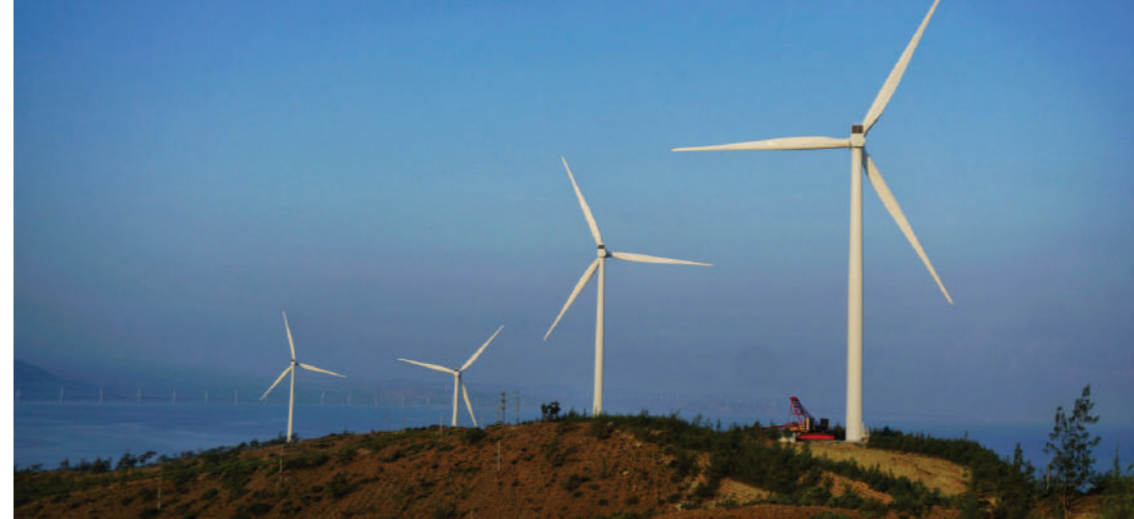
AC Energy continues to increase its renewable energy portfolio.
