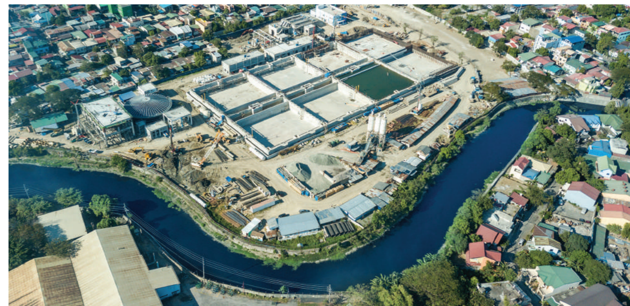
Manila Water's pipelaying project in Ilugin, Pasig is close to completion will be the largest Sewage Treatment Plant in the country with a capacity of more than 100 million liters of used water per day.
