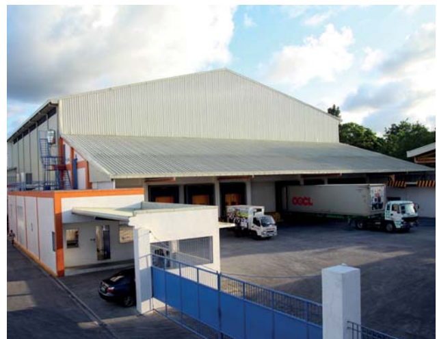
Mets Logistics: an energy-efficient cold storage facility in Carmona, Cavite, South Luzon funded by BPI.
