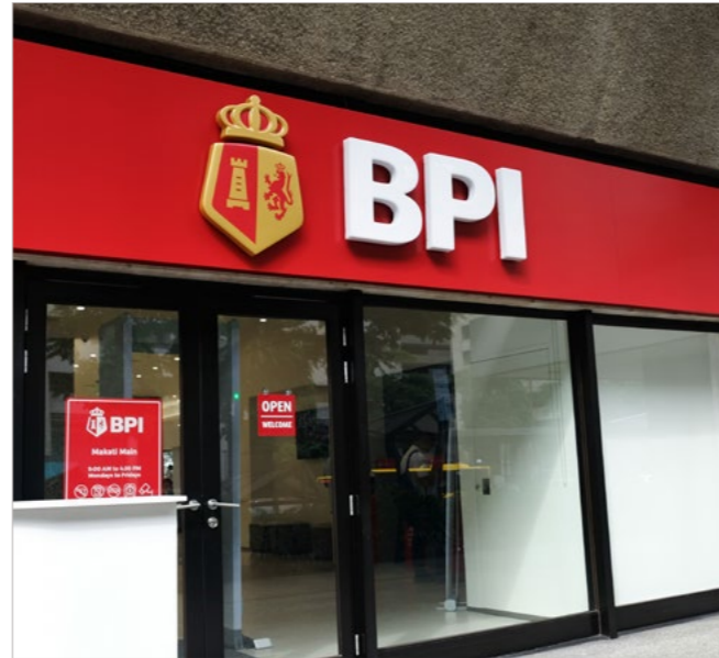
BPI completed the switch to LED lights for all its branches in the Philippines.
