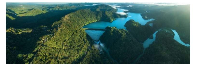
One of Manila Water's key sources of water, the Angat Dam supplies 98 percent of Metro Manila's water needs.
