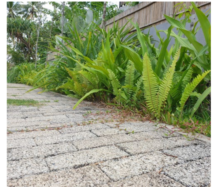
Ayala Land converts clean and dry plastics into ecopavers for use in its developments such as the Lio Estate in El Nido, Palawan.
