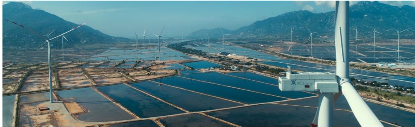
Located in South Central Vietnam, the Ninh Thuan wind farm is the second wind project in Vietnam utilizing GE Renewable Energy's Cypress turbines.
