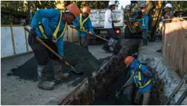
Manila Water conducts pipe laying activities to better serve its customers.
