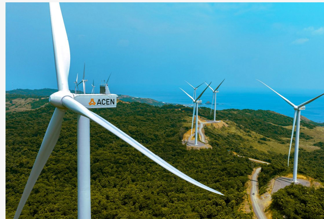
The 160-MW Pagudpud Wind in Ilocos Norte, Philippines, slated to be the biggest wind farm in the country, is the third wind farm of ACEN in the province. It is set to begin commissioning by 2023.
