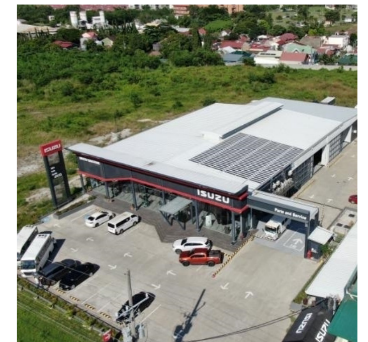
Isuzu Bacoor installed solar panels for on-site renewable energy use.
